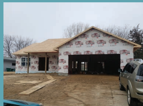
Denali Custom Homes is making great progress on the rebuild.
